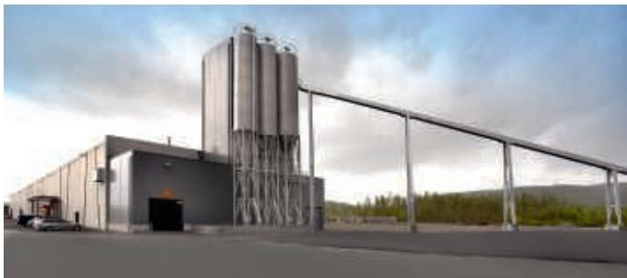
Tower plant with 2 – 2250 litres mixers for production of railway sleepers.
