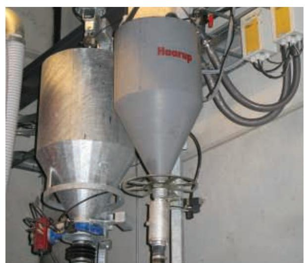
Slurry-colour and water weigh hopper with inlet and outlet valves.
