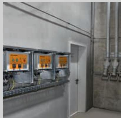
The Haarup Silo Control ensures against excess filling and excess pressure in the silo.
